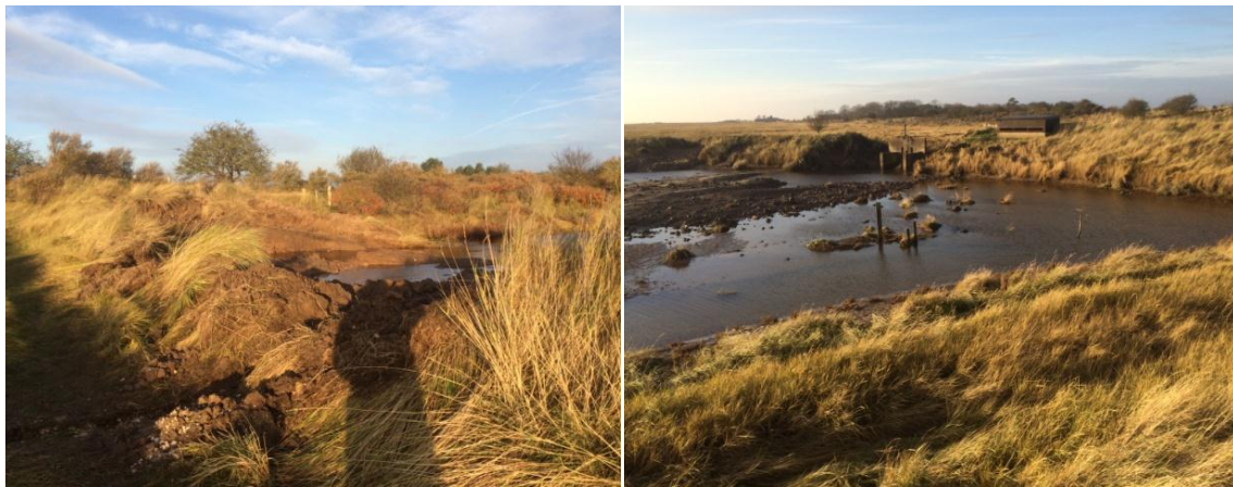
Breach point in Bulldog Bank Sluce
