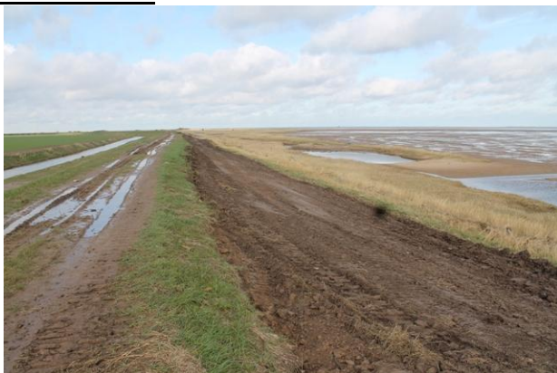
Limited repair works completed by Birse in Feb 2014
