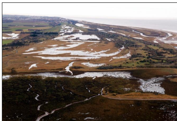
Bulldog Bank breach – Photo Taken by C J Helicopters
