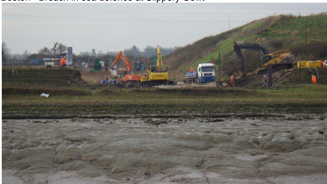
Boston - Breach in sea defence at Slippery Gowt
