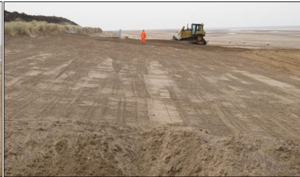
Mablethorpe emergency works
