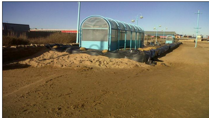
Damage to the Flood wall
