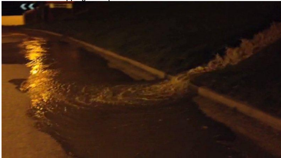
Susworth - Overtopping of steps on flood bank
