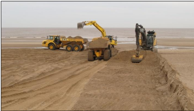
Mablethorpe emergency works
