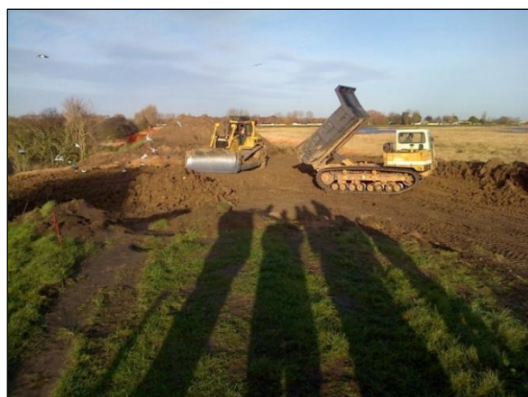
Tetney Marsh breach repairs – 20.12.13
