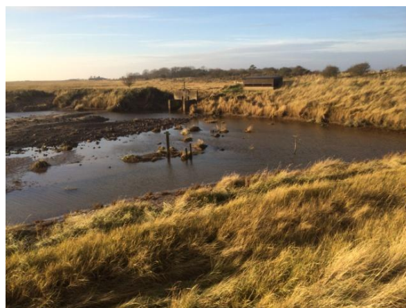
Secondary bank with sluice
